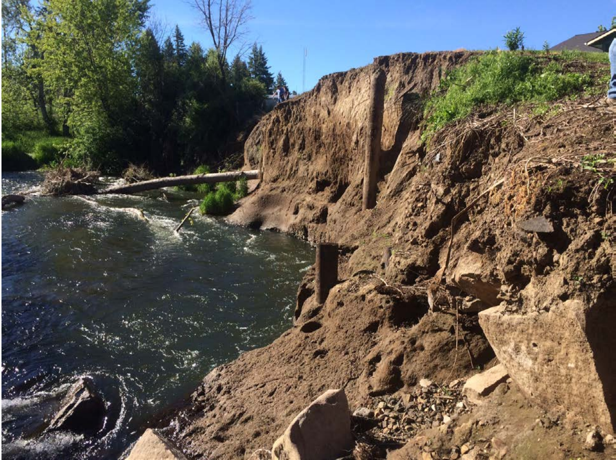
Figure 3. Silt bluff upstream of the levee tie in point.
